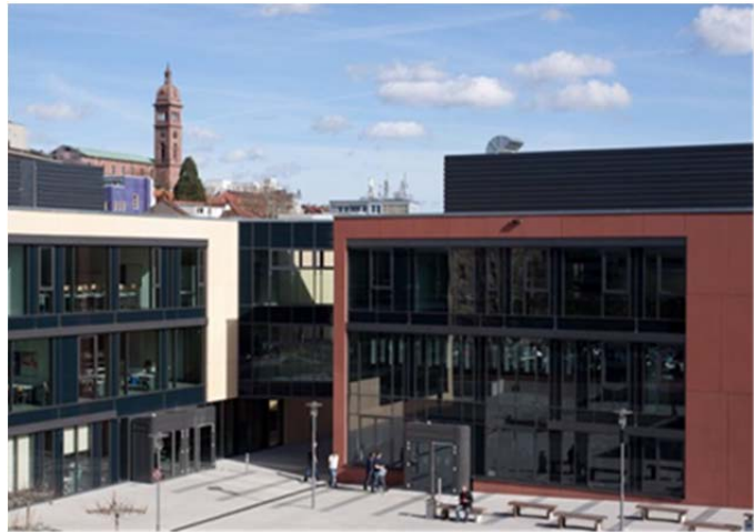
Figure 4: Pilot Project by BAM Deutschland AG
